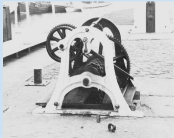
Fig. 11 Lock gear at Glasson Dock, made at Phoenix Foundry (Price 1983: 52)
