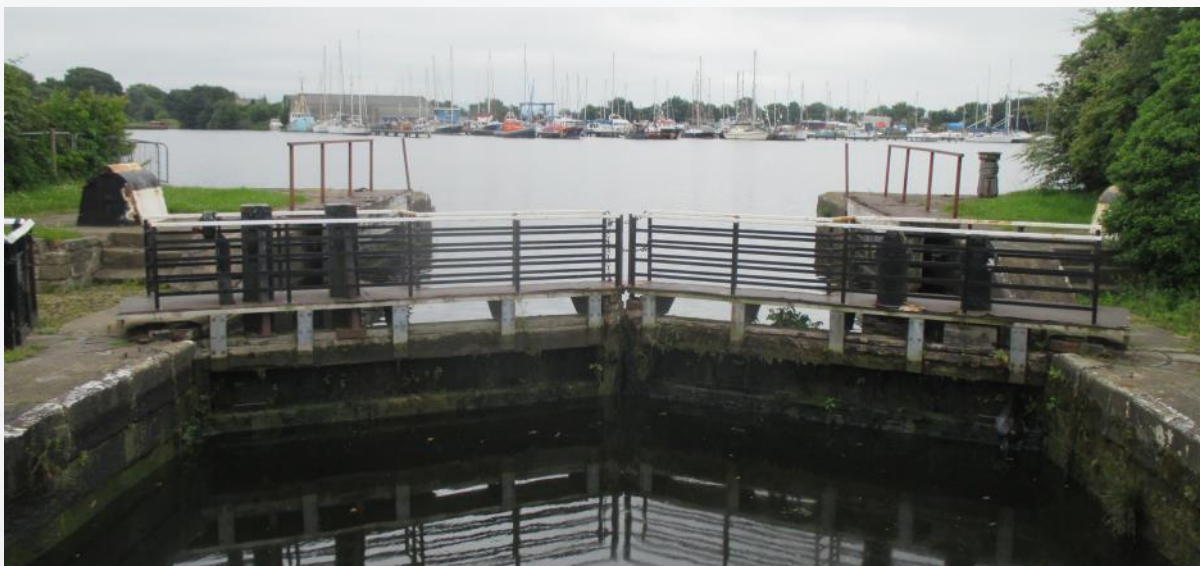
Fig. 23 Lock of Glasson Dock which leads to the canal basin. The locks have solid masonry walls with a modern swing bridge across.
