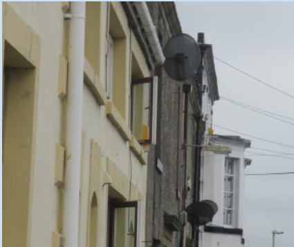
Fig. 30 Satellite dishes along front elevation.
